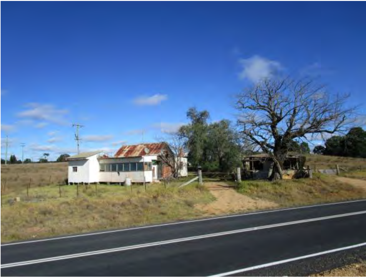
Plate 51. View of timber slab hut clad with fibro.
