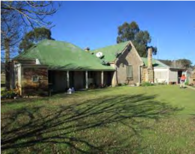
Plate 44. Rear view of Wandoona Homestead.
