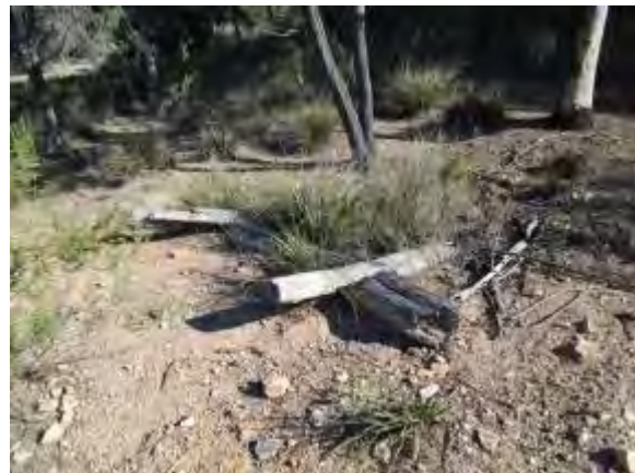
Plate 10. Collapsed post and rail fence.
