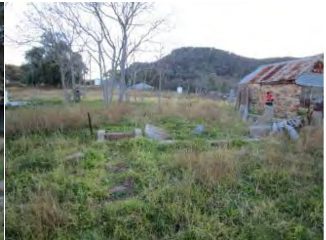
Plate 41. Cement foundations of Hillview.
