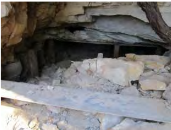
Plate 2. The timber reinforced roof of the Mine Adit.
