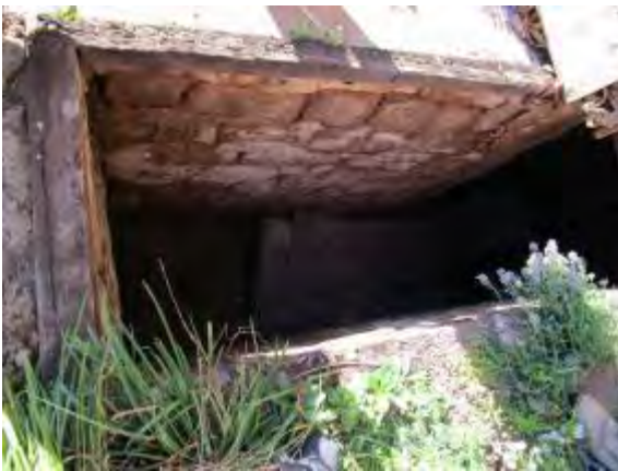
Plate 46. Sandstone lined cellar.
