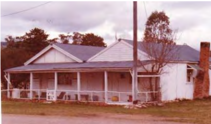
Plate 69. 1985. Former butcher and garage (Source: Gai McDermott 2012).
