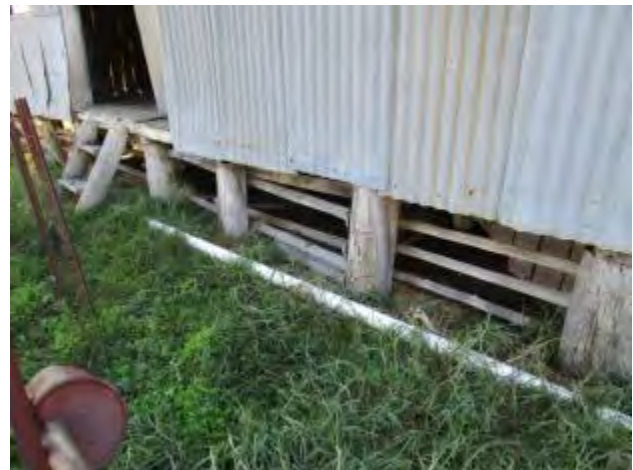
Plate 30. Raised shearing shed with room to hold sheep underneath prior to shearing.
