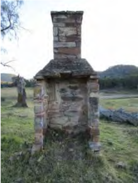
Plate 37. View of the fireplace from the old cottage.
