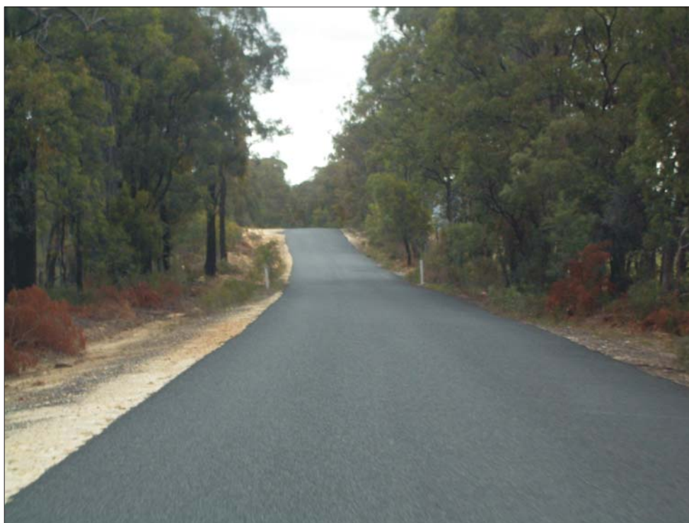
Plate 8 Ulan-Wollar Road - Looking East through a Tree-lined Section of the Road
