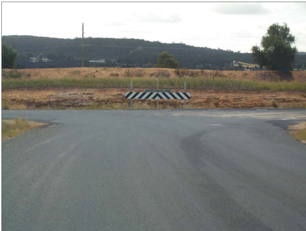
Plate 6 Ulan-Wollar Road - Looking West at Intersection with Ulan Road
