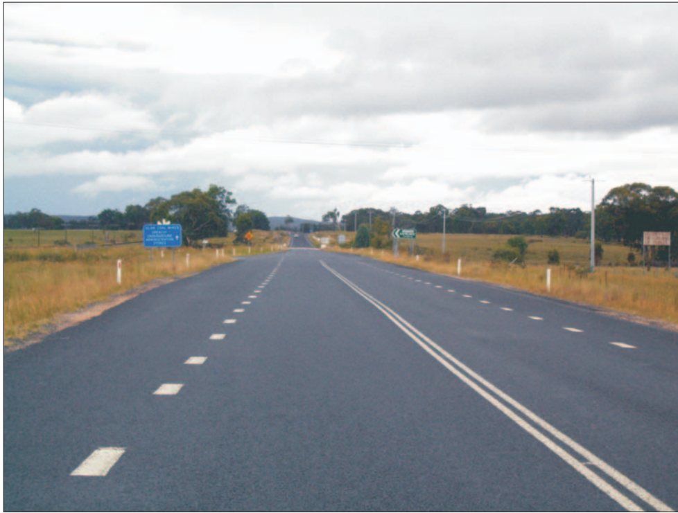
Plate 3 Ulan Road - Looking North-east at the Intersection with Ulan Township
