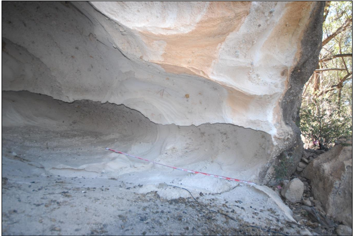
Figure 4.37 2014 (flash light) image of the southern end of the WCP152 rock shelter, showing the eroded, protruding, and fragile nature of the lower edge of the remaining art panel support. Scale is 2 m. Note vibration monitor on rock floor.
