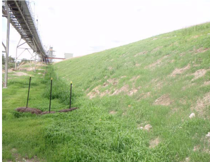
Figure 7: Hay Bales in Water Catch Drain
