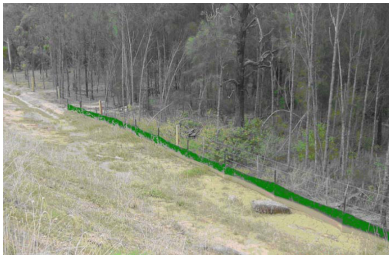
Figure 6: Example of Sediment Fencing
