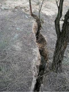
Fig. 4.5 Photographs of Surface Cracking above BSLW1 at the Blakefield South Mine
