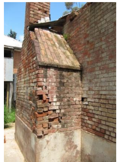
Figures 3.48-3.51 External elevations after repair and propping works. (GML 2012)
