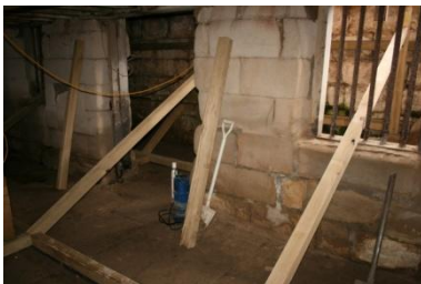
Figures 3.44-3.47 Interior views of Kitchen Wing including original stone walls (after removal of modern linings), fireplaces in kitchen (west elevation), first floor accommodation and Cellar/Basement stonework after propping. (GML 2012)
