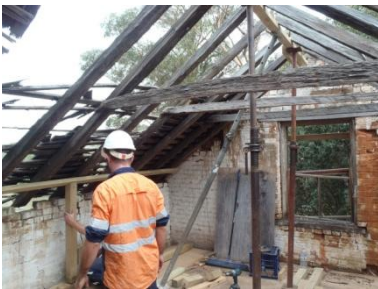
Figures 3.52-3.55 Interior views of Servants' Wing after clearing out and propping including supports to brickwork and structural framing at ground and first floor levels. (GML 2012)
