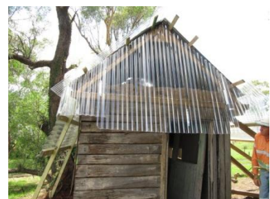
Figures 3.56-3.59 Butcher's Hut after restoration of slabs, propping and new weather protection. (GML 2012)
