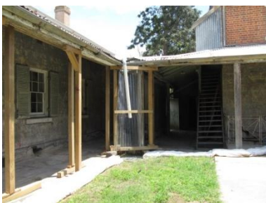
Figures 3.28-3.31 Front and rear elevations of New House with removed fabric (for safe storage in building), propping of verandahs and detail of junction with Kitchen Wing. (GML 2012)
