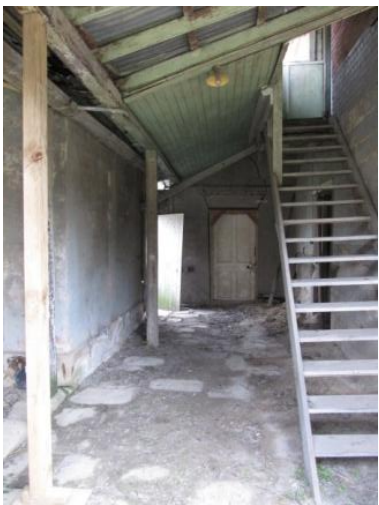
Figures 3.36-3.39 External views of east and south elevations of Kitchen Wing including junction with northwest corner of New House, stair case to first floor accommodation and salt-damp attack in ground floor stone walls. (GML 2012)
