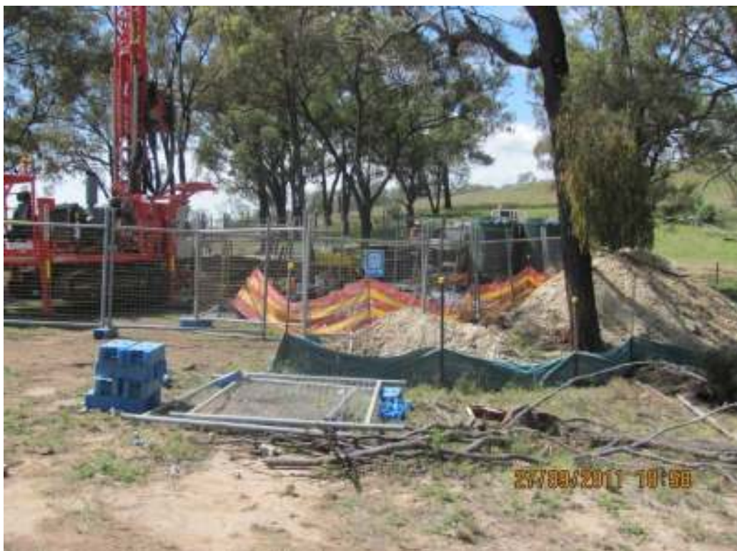
Plate 8 – view of the active United Drill Site UG238. Note the top soil is separated in the closest stockpile and has been separated from the underlying soil. Also, United advised that the fallen branches from the drill pad have been collected and will be re-placed across the drill pad following completion of drilling activities.
