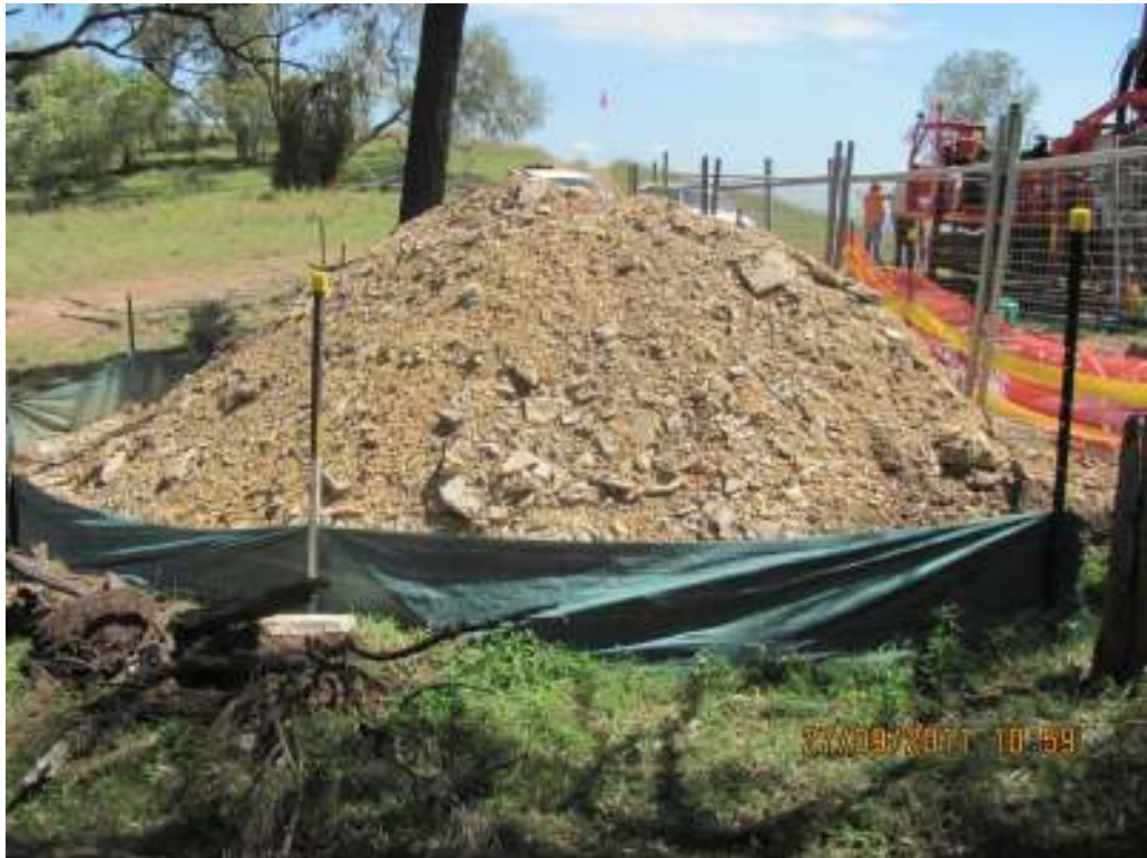
Plate 9 – view of the active United Drill Site UG238. Note the use of sediment fences
