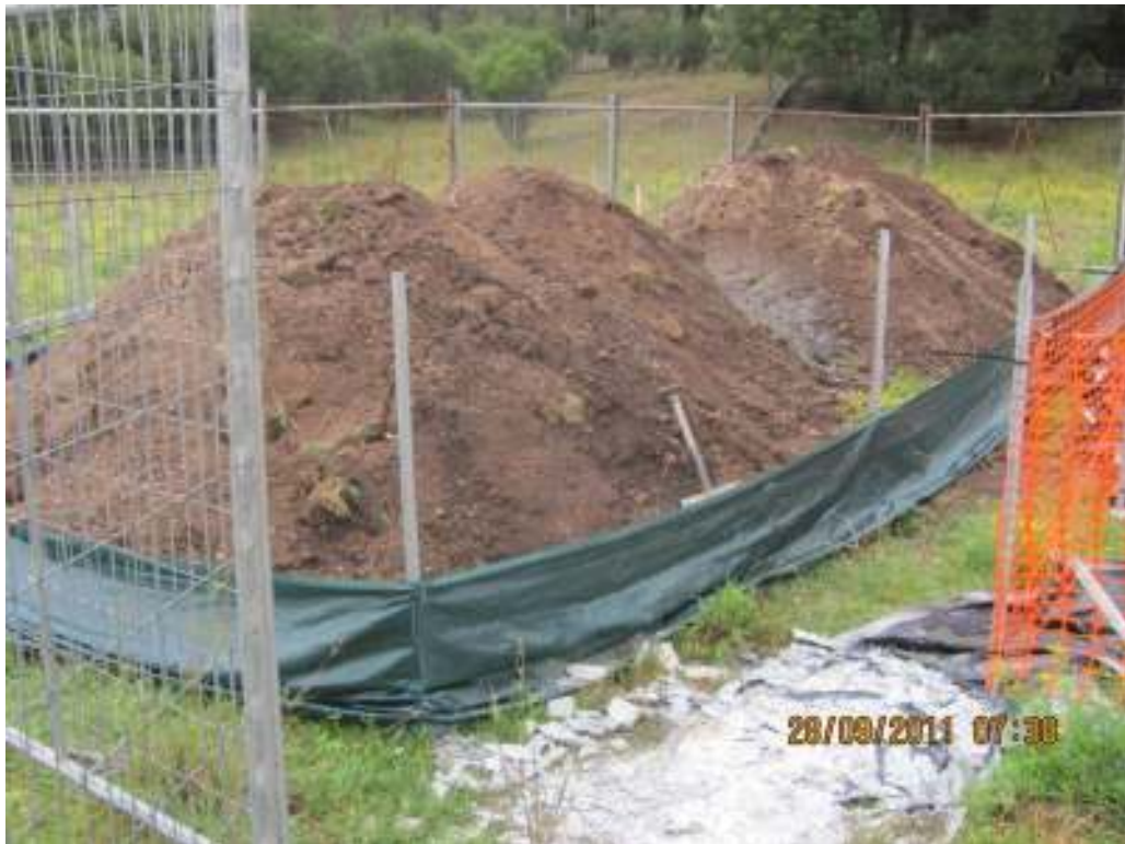
Plate 14 – view of the active Wambo Drill Site (not within A444). GSSE observed that the top soil was stockpiled separately and sediment fences were being used.
