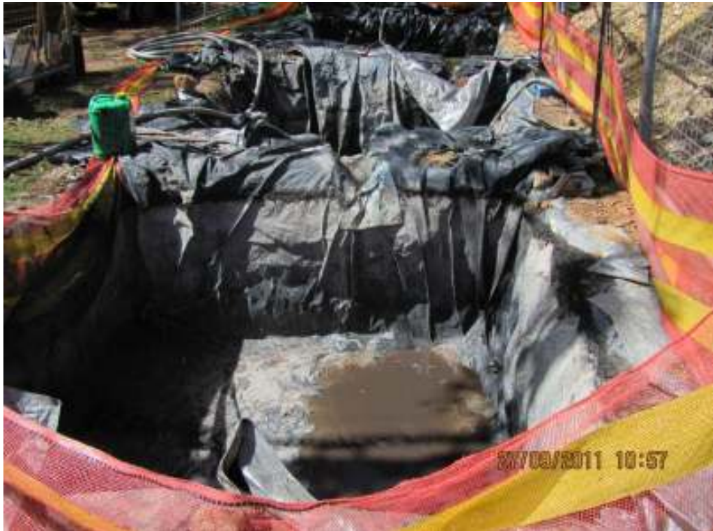
Plate 7 – view of the three sumps at active United Drill Site UG238. Note the use of plastic liners.
