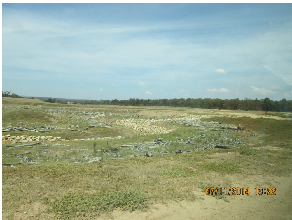
Plate 14 Rock structures within the North Wambo Creek Diversion Channel
