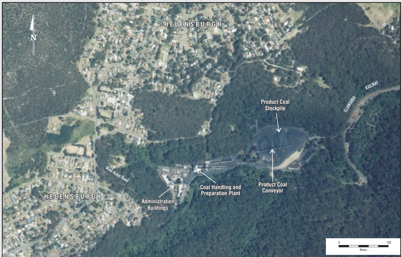
Metropolitan Colliery Major Surface Facilities Area
