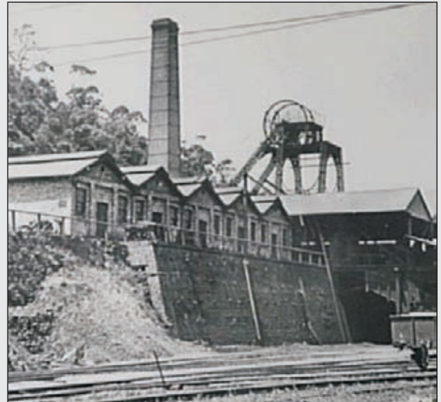
Historical Photograph - Metropolitan Colliery
