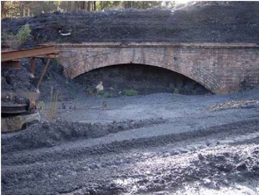
Figure 26. The viaduct that carried the colliery siding over the main line. The parapet has been removed, and the bridge buried in coal stockpile material.
