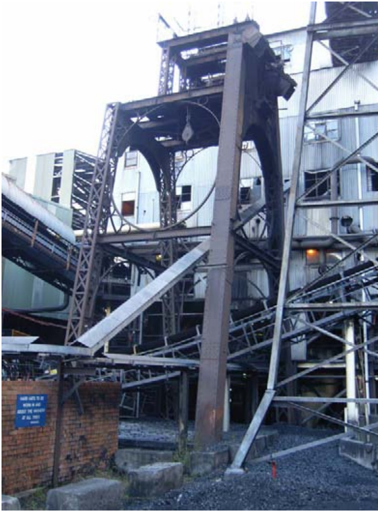
Figure 7. Shaft No. 1 headframe. The stumps of the cut-off brace legs can be seen to the right and the top section. Washery behind. 2007.
