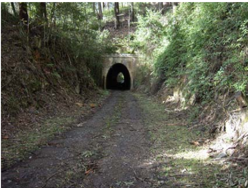
Figure 28. Rail tunnel No. 5 (aka Lilyvale No. 1), in the northern section of the Metropolitan lease area, showing single-track width and ovoid brick form.
