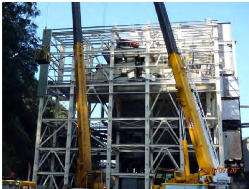
Plate 2 CHPP Installation of Noise Insulation
