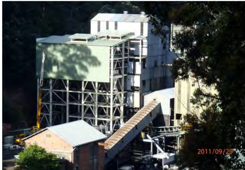
Plate 1 CHPP Installation of Noise Insulation
