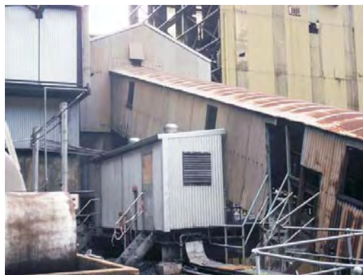
Plate 4. MD1 after enclosure and insulation
