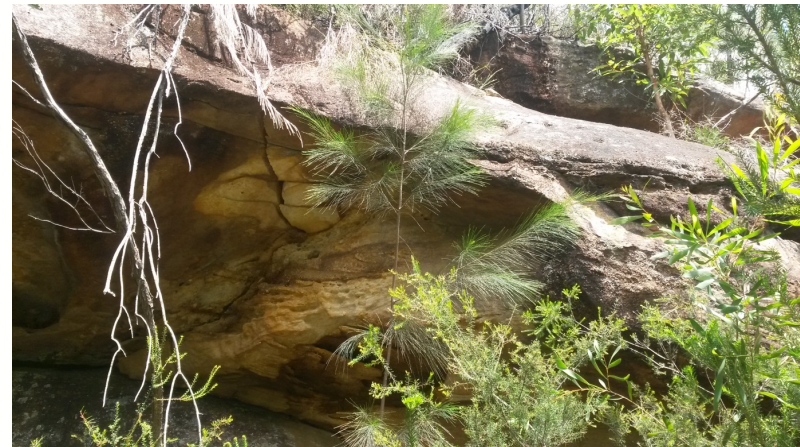
Plate 1 Tension Crack on Cliff Face at Site COH2 (Looking West toward Cliff)
