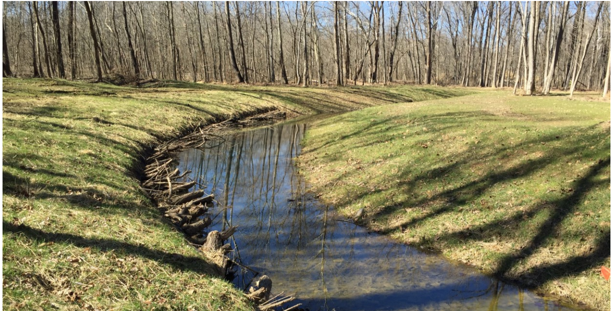
Willow tree cuttings were installed as toe wood in three locations along the restored stream channel to provide high-level habitat for both aquatic and terrestrial fauna. Here, woody material purposefully protrudes along the outside bend of the Big Creek channel.
