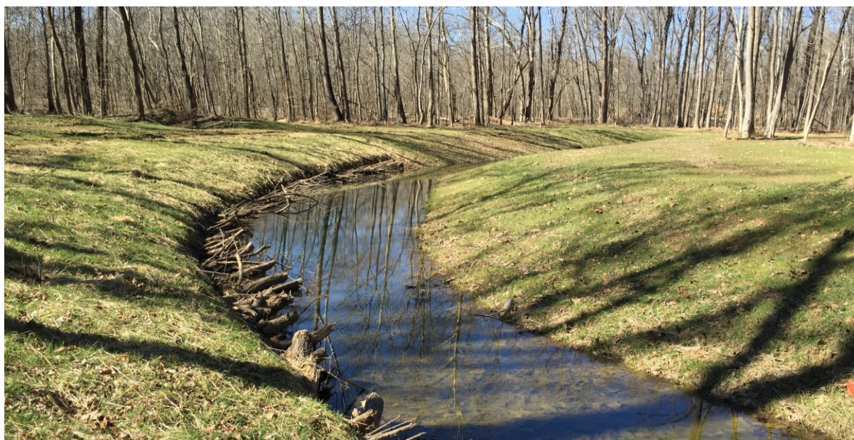
Willow tree cuttings were installed as toe wood in three locations along the restored stream channel to provide high-level habitat for both aquatic and terrestrial fauna. Here, woody material purposefully protrudes along the outside bend of the Big Creek channel.
